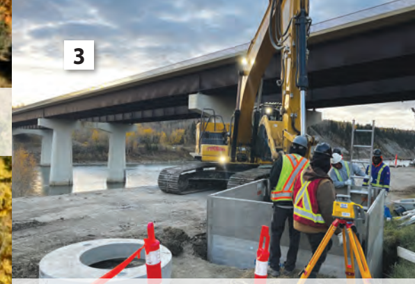
Installing a catch basin, Prospector's Point Road Rehabilitation.
