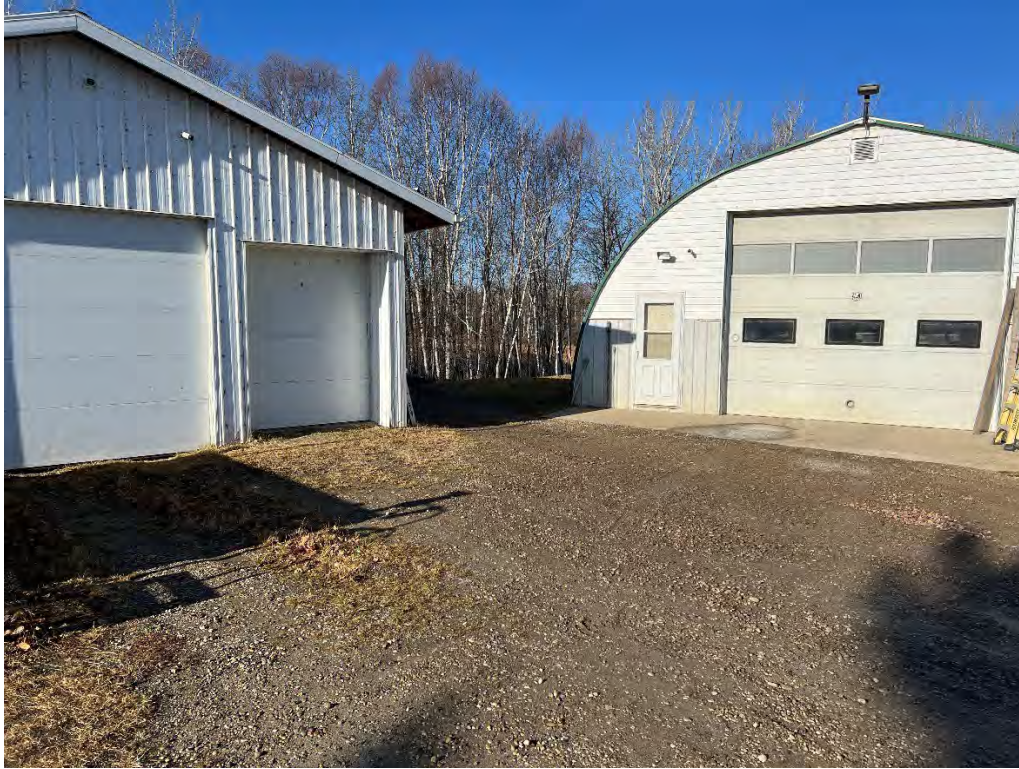
Shop and Storage Buildings.
