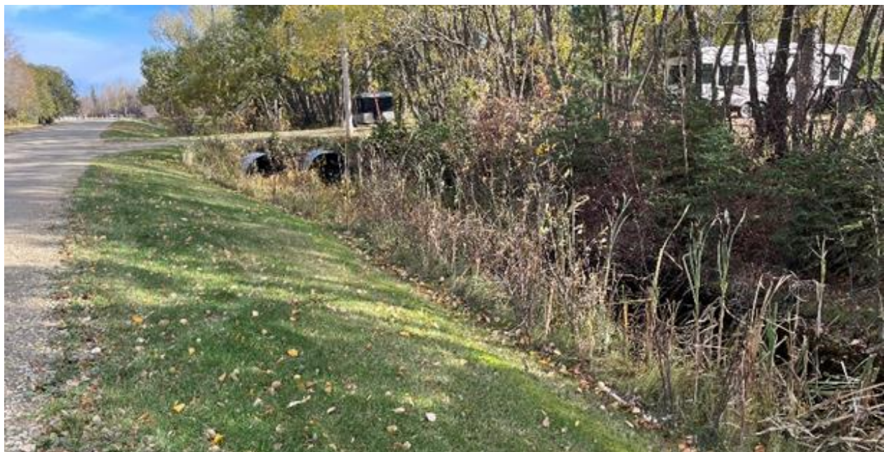
Lot 17 Driveway Culverts
