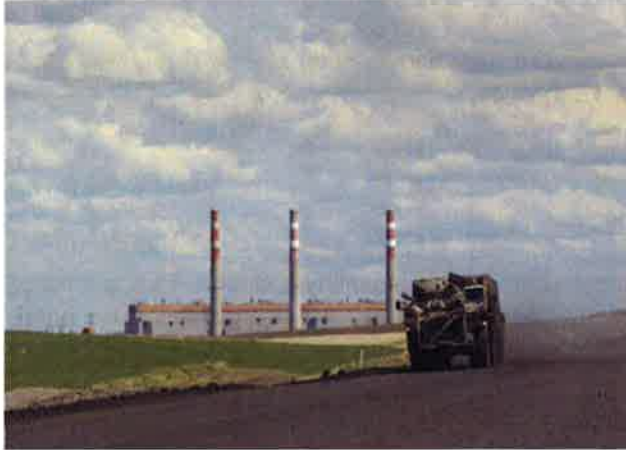
Haul Road near Sundance Generating Plant: Courtesy of TransAlta
