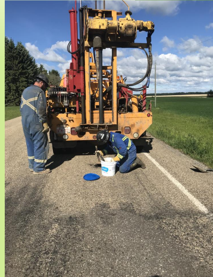
Photo: Drilling subcontractor conducting soil suitability drilling
