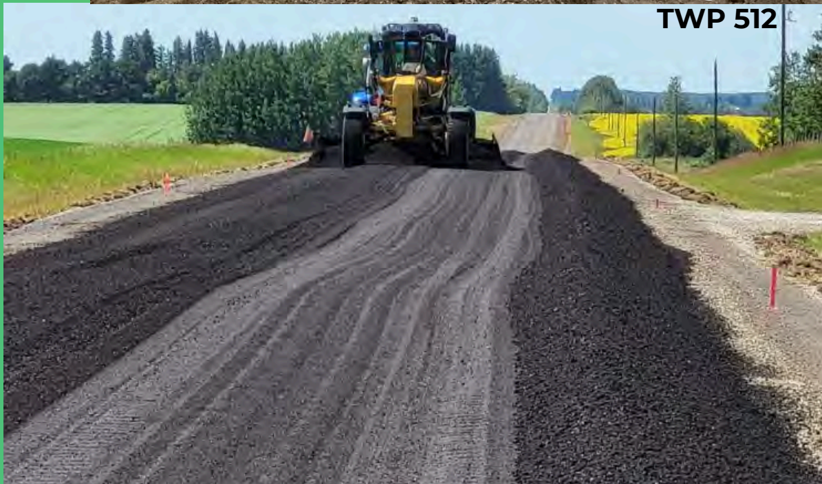
2024 Surfaced Road Reconstruction Program
